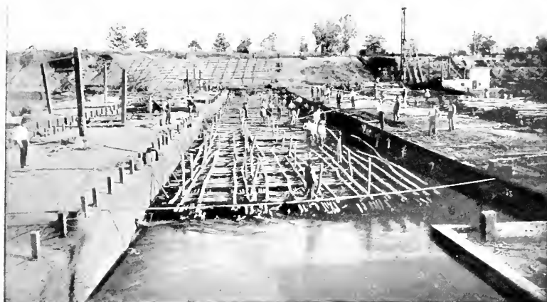
SPUR CONSTRUCTION ; GREENVILLE, MISSISSIPPI.
